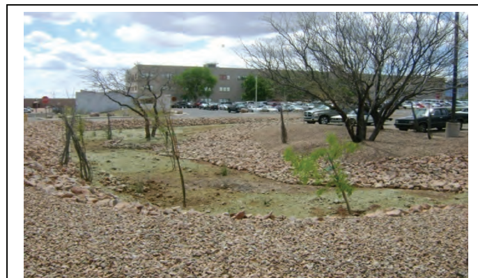
Detention basin to detain and recharge storm-water - Ft Huachuca
